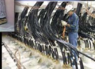
**3** Beam tubes transport laser light to the target chamber.
